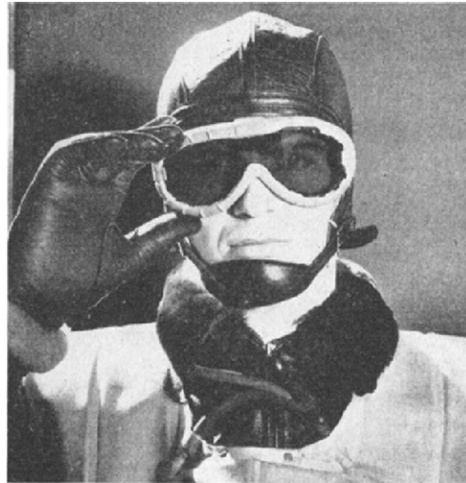
Fig. 1. New dark adaptor lenses, developed by the Medical Research Section of the U.S. Navy's Bureau of Aeronautics. Three plastic polaroid goggles, with red lenses, enable pilots to work in the 'Ready Room' under full illumination and thus eliminate the 20- to 30-minute period usually spent in a dark room to condition their eyes for night flight (official U. S. Navy photograph).
